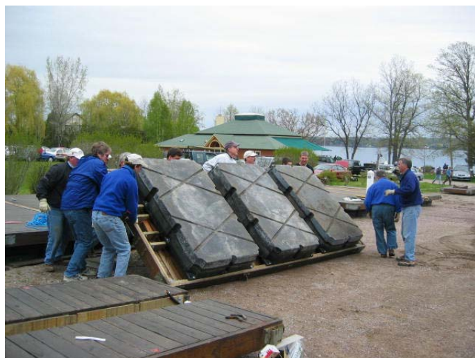
Dockwork in Progress—Spring Workday 2005
